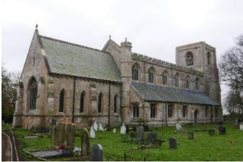
All Saints', Bennington, medieval with Victorian restoration.
