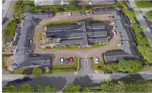
Waterpark Hall, United Reform Church
