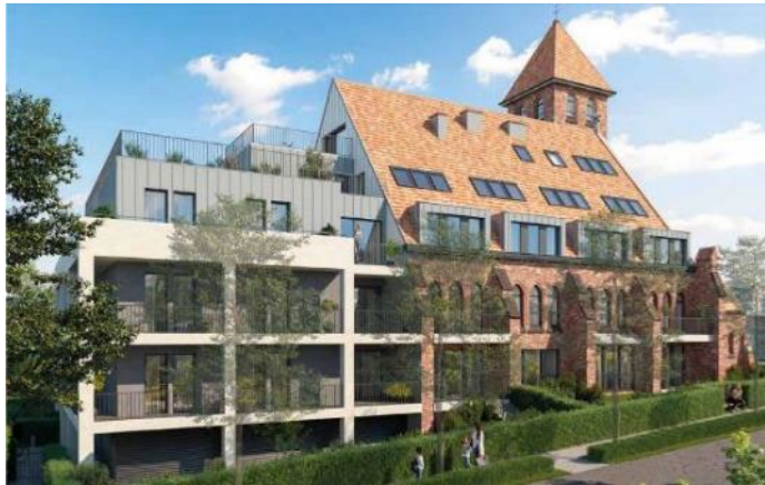
L'Eglise Saint Joseph, Parvis Chantecler, Brussels Conversion and extension into 14 apartments Of particular note here is the extension, and the balconies cut into the sides of the nave and roof
