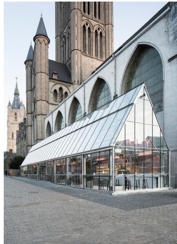
Figure 6 Church of St Nicolas with the temporary addition, a conservatory. Photo by RAY
